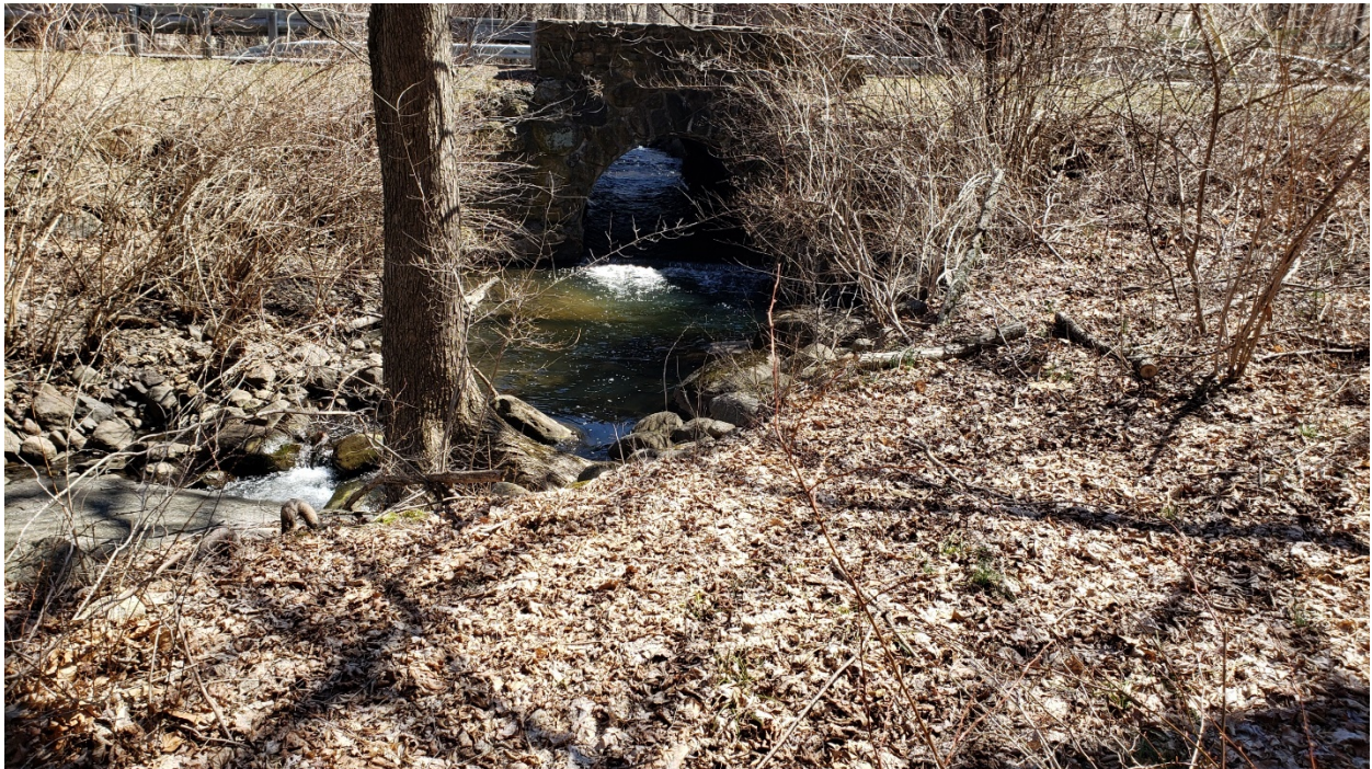
3/26/2019 Tributary 5 inlet in northeast portion of the Property
